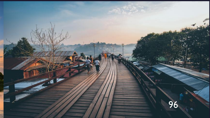
Uttamanusorn Bridge, Kanchanaburi
