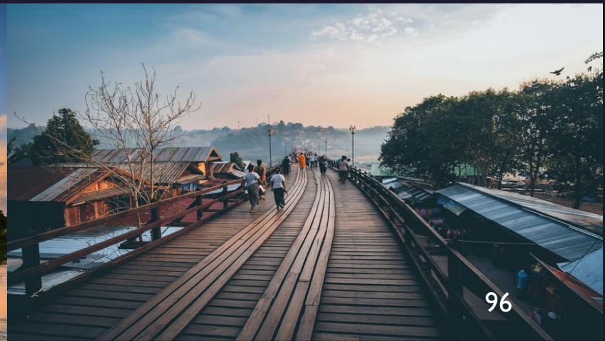
Uttamanusorn Bridge, Kanchanaburi
